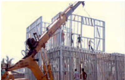
Easy installation at site Wall Panel assembly erected at one go.
