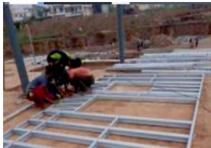
Easy installation at site Wall Panel assembly erected at one go.
