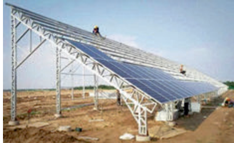
Mounting Frame in Cold Formed Section for Solar Panel Arrangements Ref. FrameCAD Website
