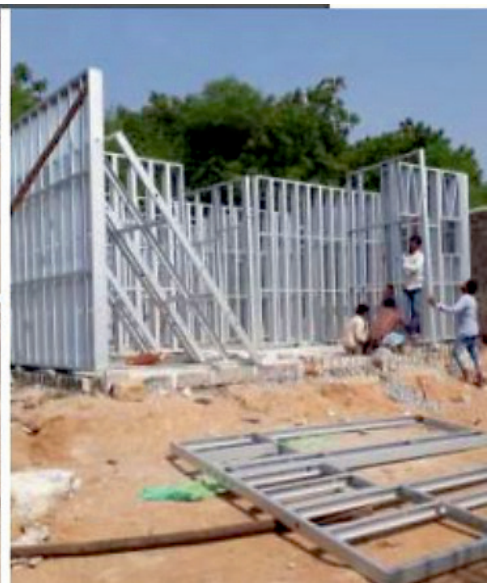
Wall Panel with Cold formed steel sections
