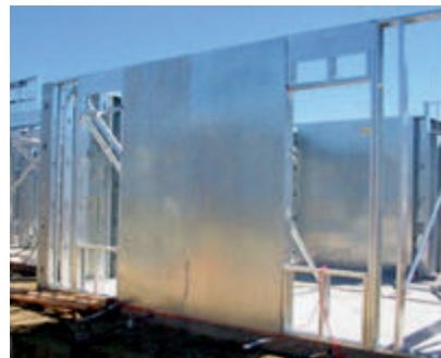
Steel Sheet in Sheathing in Shear Wall Panel Ref. Thin Walled Structures, Research Paper, Elsevier Journal, Volume 75, February 2014.
