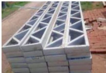
Wall Panel with Cold formed steel sections
