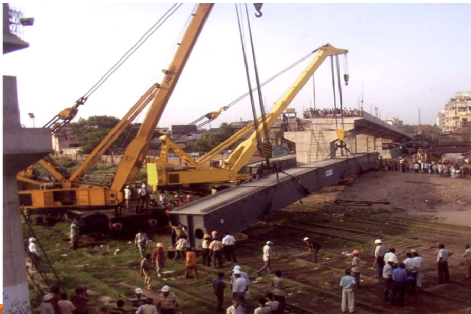
Steel box mandatory span being erected – Lock gate crossing
