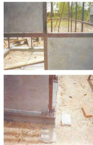
**Connection of SHS with Ferro cement panel**
