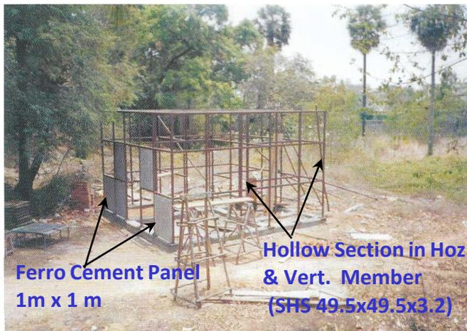
**Structural Frame & Ferro cement panels while Installation**
