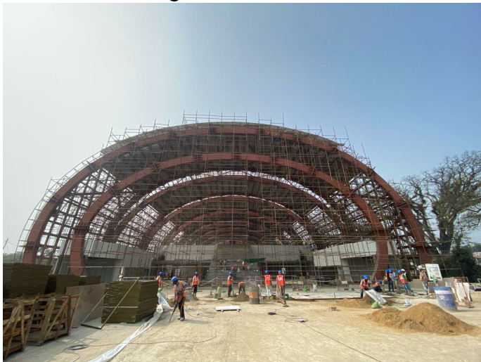
Fig 3: Full frontal view of the structure
