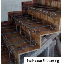
Formwork for stairs - Formwork for stairs consists of stringers, sheets, joists, bearers and vertical post.
