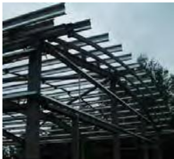
Purlins in the steel framing
