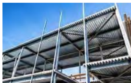
Metal decking for slabs
