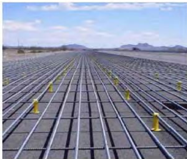
Fig.5: Continuously Reinforced Concrete Pavement
