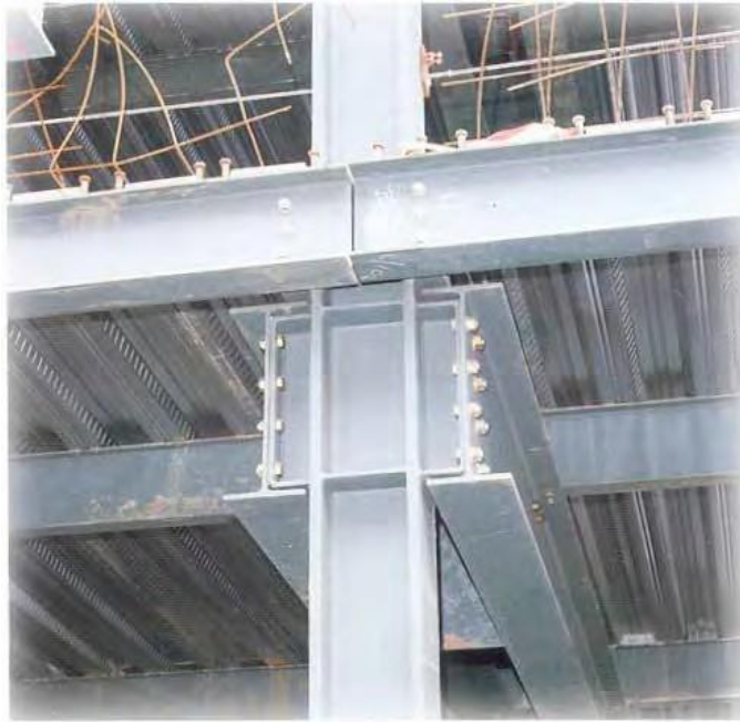
Fig.2: Easy Connections Using Parallel Flange Sections
