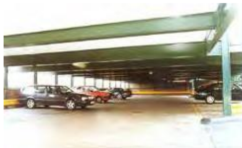
Fig. 9: Car Park with PF Sections
