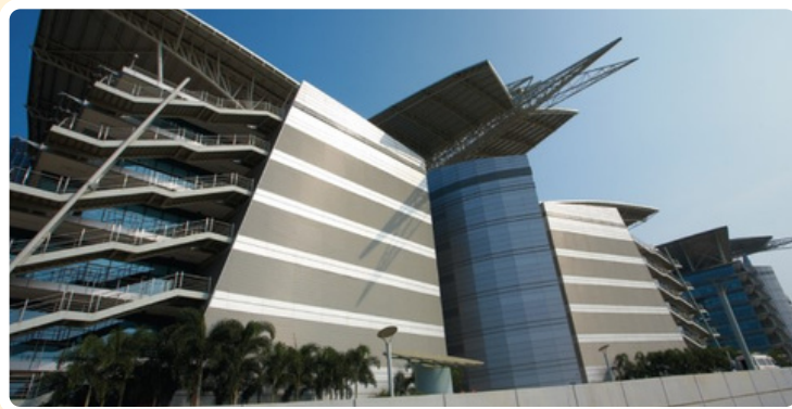
Fig 44 : TCS Technopark Building Chennai
