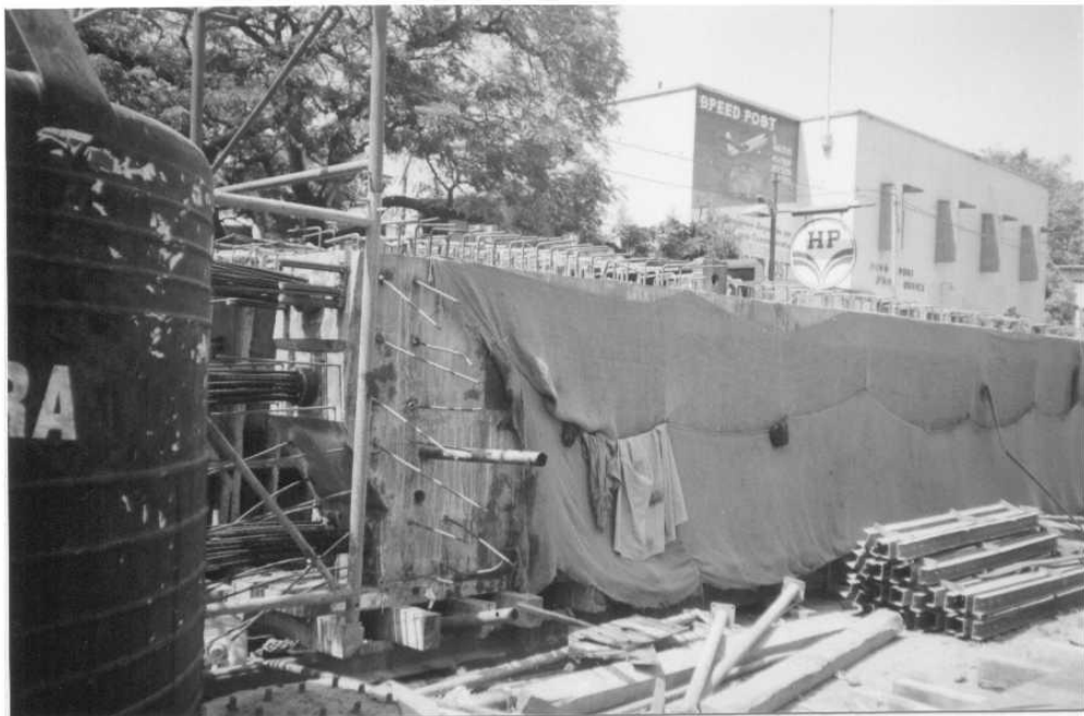
Fig. 1 Flyover construction – The Indian way
